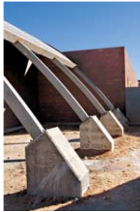
Bringing engineering laboratories under the same roof in the 20,000-square-foot Aerospace Experimentation and Fabrication Building (AXFAB) mimics the efficiencies and integrated design practices of today's industry and will help build synergy between engineering students and faculty, and among faculty from various programs.
