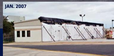
and home to more than 120 employees, was hit so hard by the storm that its internal steel frame bowed inward. In an eerie coincidental turn, the storm ripped away pieces of the building to reveal a “Merry Christmas” message from 1986, spray-painted on a length of its steel beam.
