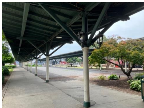
The tracks being made into a public garden
