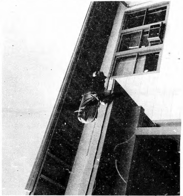
TWELVE WORKMEN WERE REPORTED LOST LAST SATURDAY WHEN THE ENGINEERING BUILDING WENT DOWN IN A HEAVY STORM.
