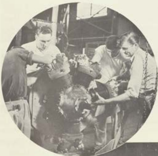
Students learn piston engine theory and construction by dis-assembling engines.
