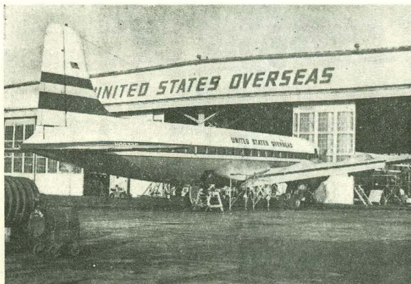
HOME BASE — United States Overseas Airlines' operates out of the Cape May County Airport, Wildwood. Its 15 four-engine DC-6's and DC-4's receive maintenance and overhaul service here from a crew of skilled mechanics and aircraft service specialists.
