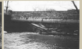
Collapse of the Ynys-y-Gwas bridge in South Wales
