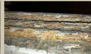
Shows the top of a tendon found in the Ringling bridge with deficient grout and strand corrosion
