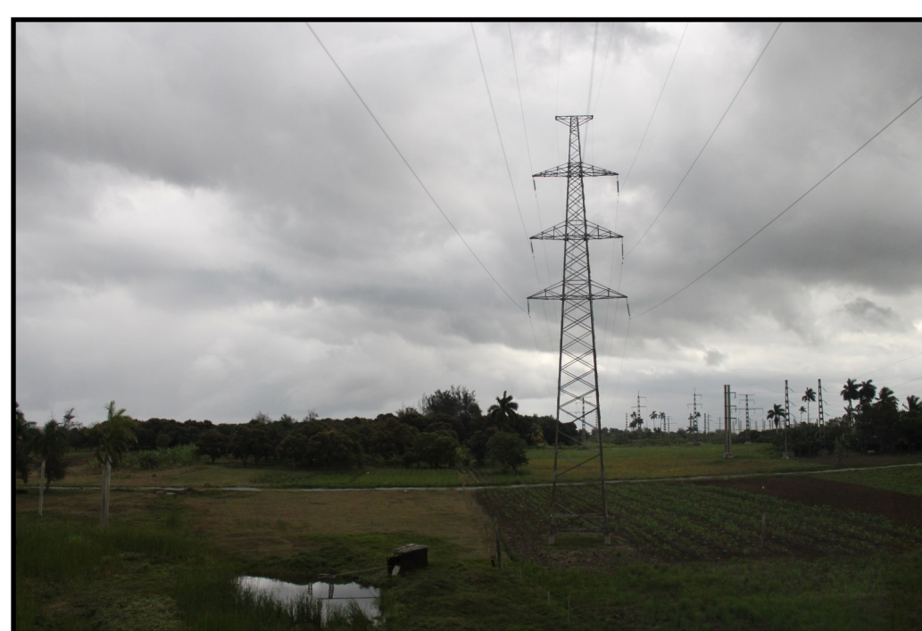
Cuba's electricity grid extends far out into the country. Most, if not all of the energy grid is above ground.
