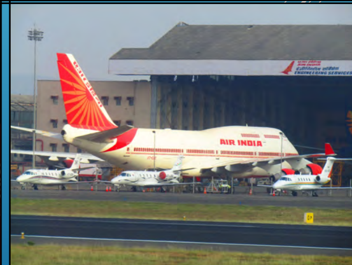
Air India Maintenance hangar, Mumbai
