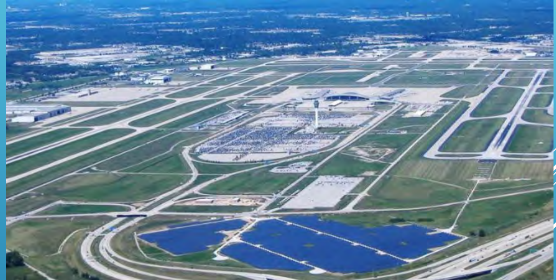
Solar farm at Indianapolis International Airport
