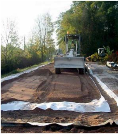
Fig. 2 An example of product re-use in road building [3].
