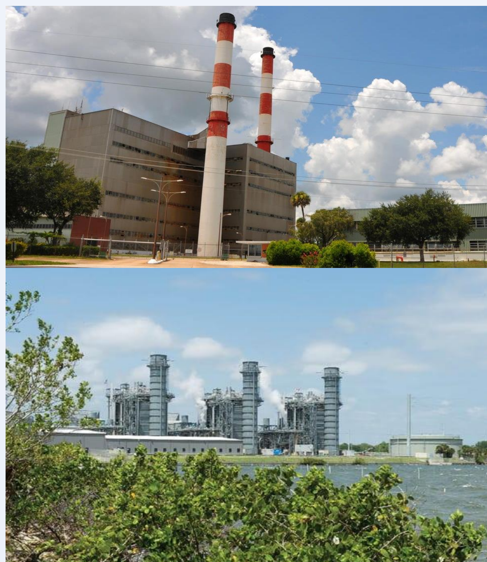
Figure 1: OUC Indian River Plant (Top) & FPL Cape Canaveral Power Plant (Bottom)
