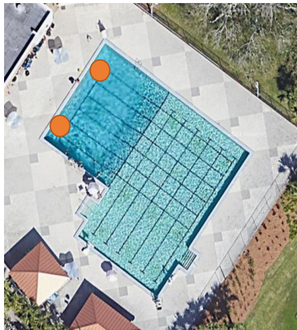
Figure 65: Pool test environment overhead (Google, 2021).
