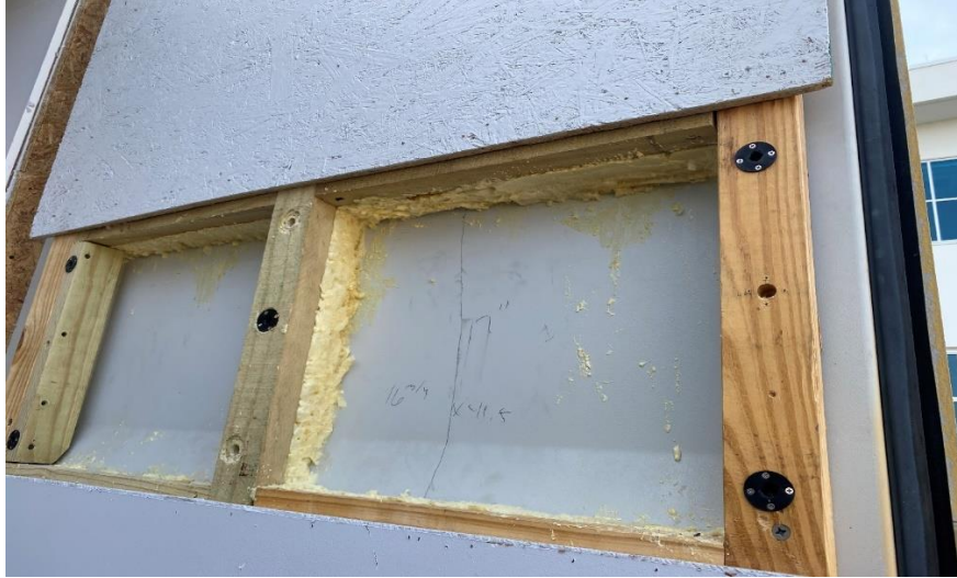
Figure 71: ACE lab exterior.
