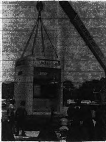
An electronic bank tower is lowered into position on the north side of the raceboat harbor to provide instant-money.
