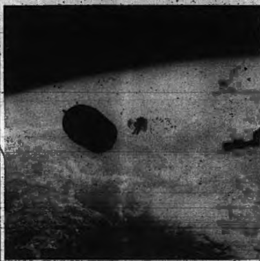
Dale Gardner files an MMU toward the Westar IV satellite prior to docking. Discovery's RMS awaits at right. Dr. Anna Fisher later used the RMS to grapple the satellite.
