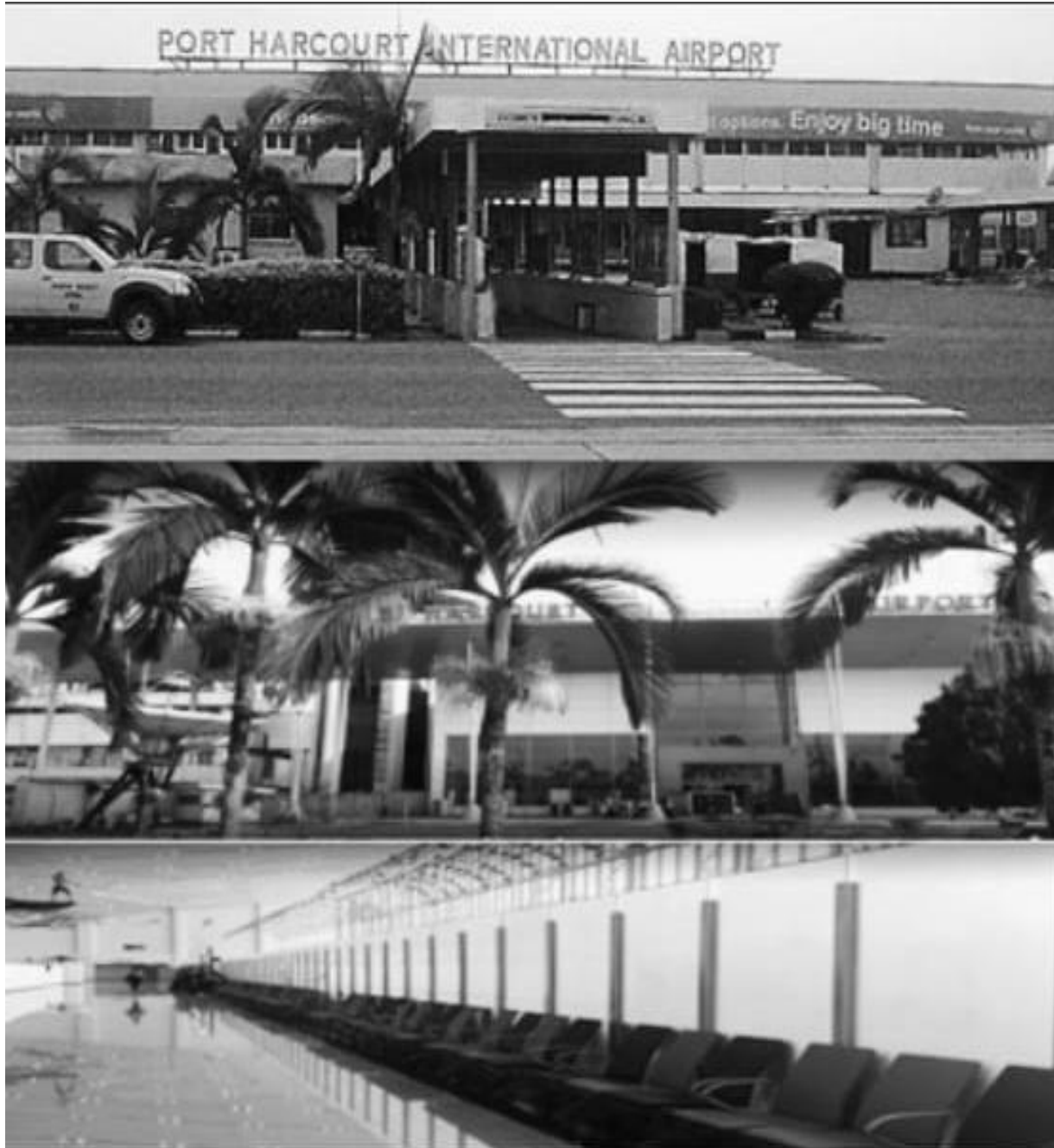
The Terminal Building after the 2013 Remodelling Exercise
