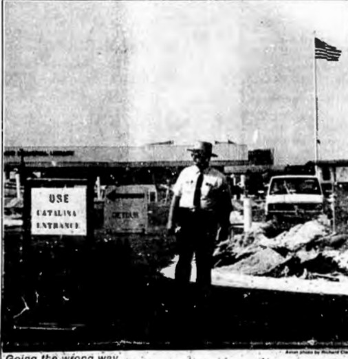
Going the wrong way...
