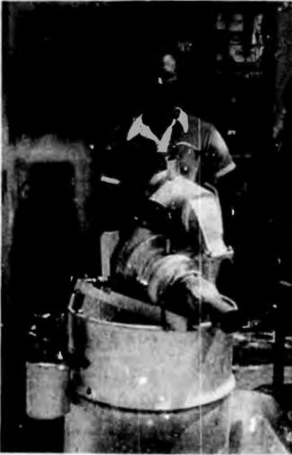
Chris Cuneo poses behind his latest creation, a centrifugal flow turbine engine. The engine, with afterburner, will produce approximately 200 pounds of thrust.
