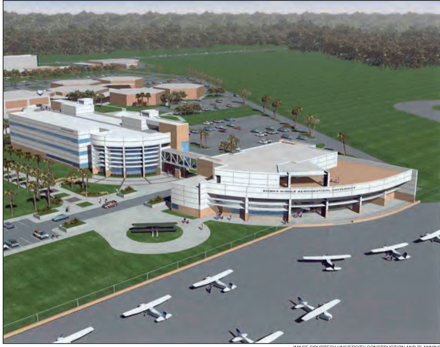
IMAGE COURTESY UNIVERSITY CONSTRUCTION AND PLANNING
