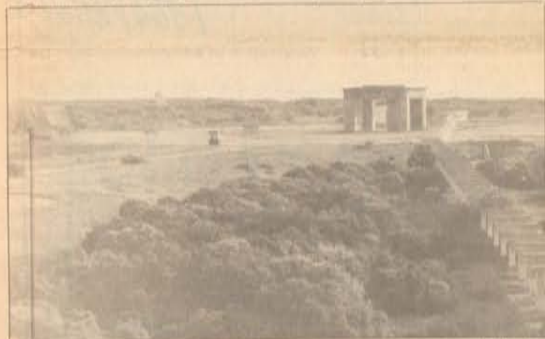
Remembering... The remaining structures of Launch Pad-34 remind us of the three astronauts who lost their lives testing the Apollo spacecraft systems. Edward White, Virgil Grissom, and Roger Chaffee died January 27, 1967.
