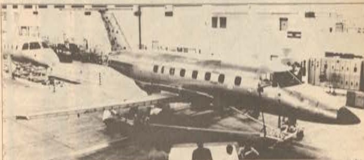
Leaving the jig... The first prototype of Embraer's CBA-123 19-seat pusher turboprop, seen here being moved to final assembly in Sao Jose Dos Campos.
