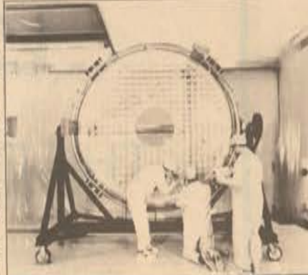
Scratched?... Technicians are seen here inspecting the polished 94-inch primary mirror prior to application of the reflective coating.
