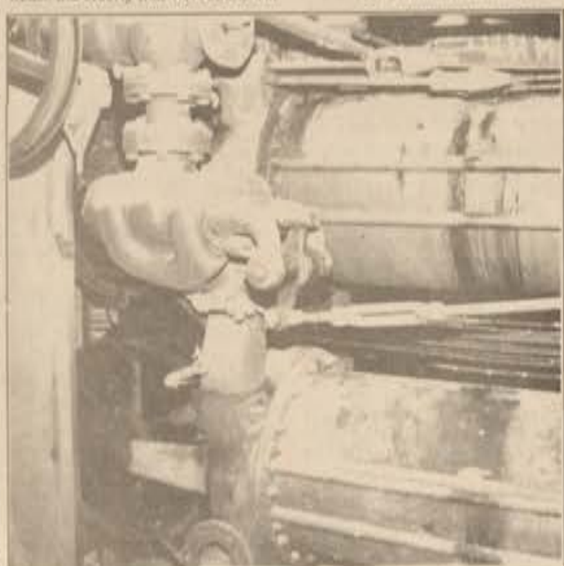
The elevator in the hotel was powered by this Steam Engine. There were only two of these engines built, and this is the only one which is still in working order.
