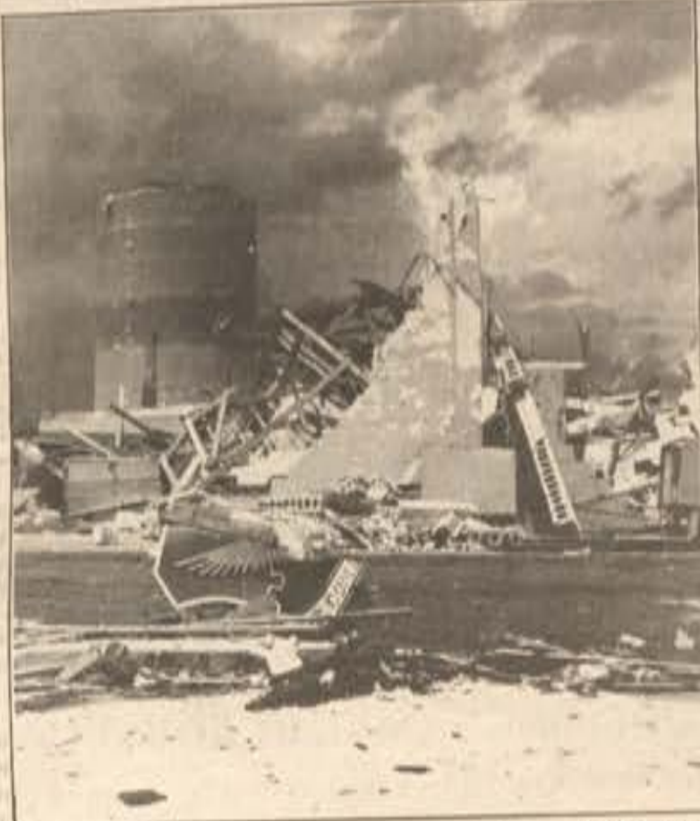
Homestead Air Force Base was destroyed by the 164 mph gusts of hurricane Andrew. Homestead AFB was at the location where the eye of hurricane Andrew hit.
