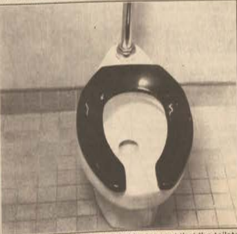
It has been decided by our resident expert that the toilets in the library are by far superior to other toilets on campus. These bad boys were build for comfort, not speed.
