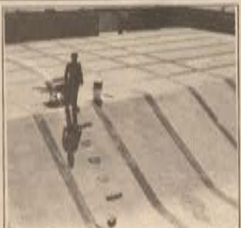
Physical plant is finishing improvements to existing athletic facilities on campus.
