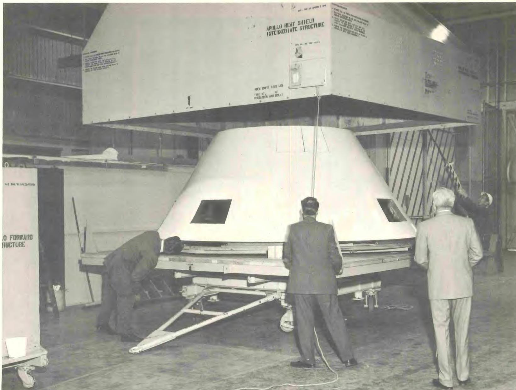
Figure 5 Shipping The Completed Crew Compartment
