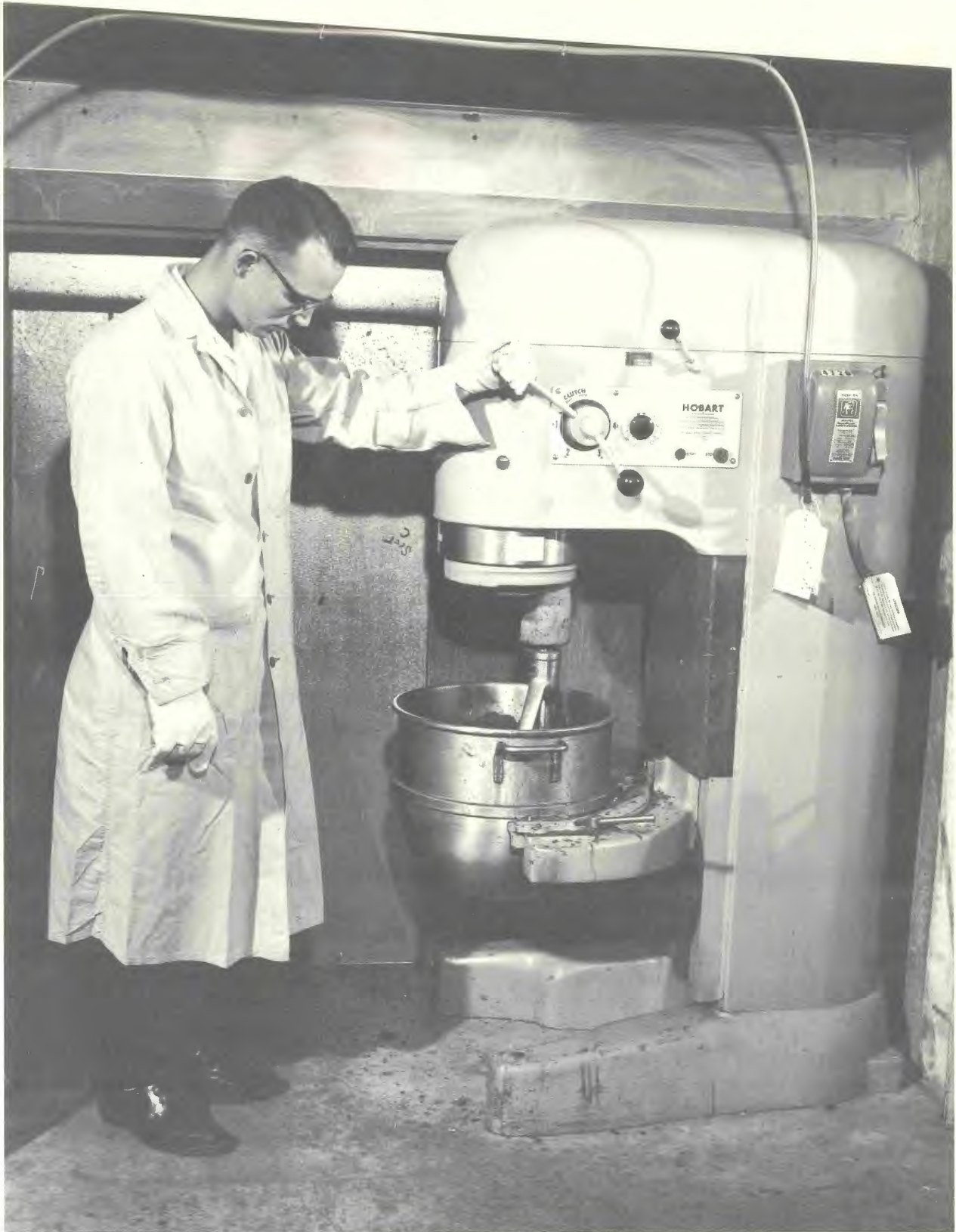
Figure 6 Mixing the Ablative Material
