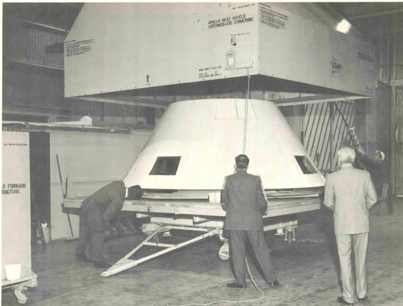
Figure 5 Shipping The Completed Crew Compartment
