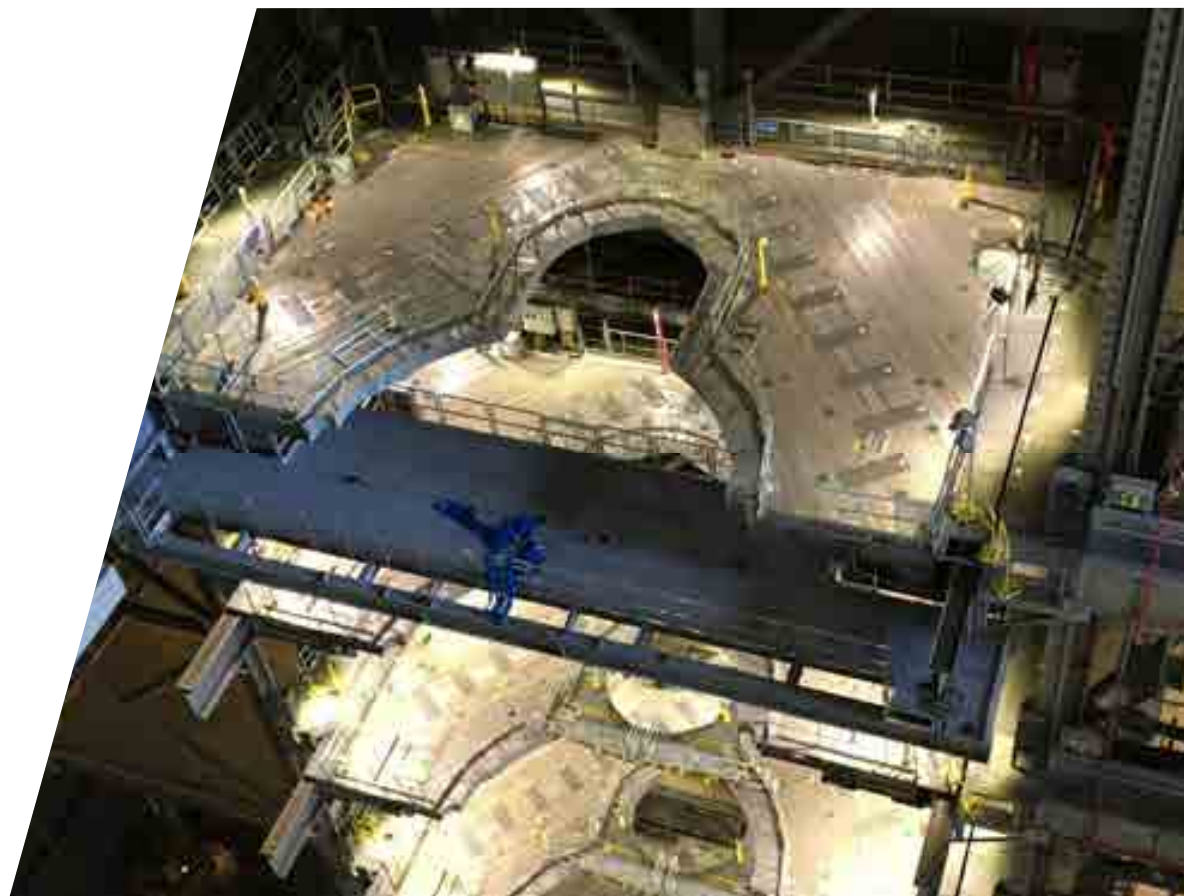
Construction Aid Platform Photo credit: RS&H/Mike Kendrick 32
